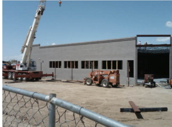
Figure 2: Walgreen's in progress
