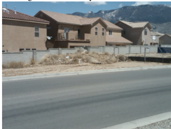
Figure 5: 9100 Holly construction area
