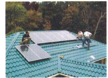
Builders installing photovoltaic solar electric system.
